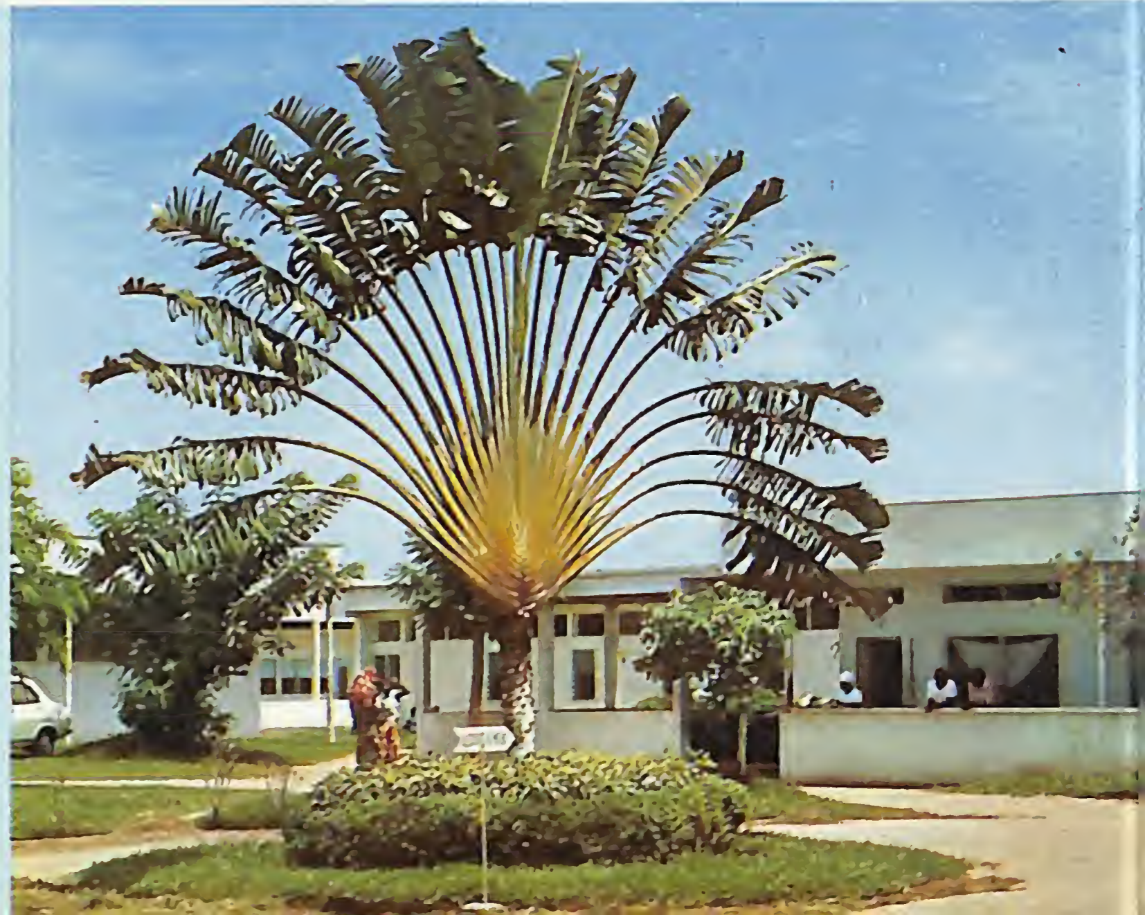
Maternity department of the Makele-kele Medical Centre.
